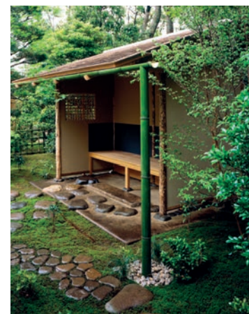
Above A simple gutter made from bamboo poles catches water running off the roof of the koshikake machiai (waiting bench).
