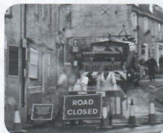
5 Repairs to streets and motorways. (4, 5)
