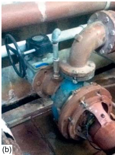
FIGURE 16.11 (a) Schematic of a centrifugal pump (from http://navalfacilities.tpub.com/mo230/mo2300161.htm ). (b) Centrifugal pump in use.
