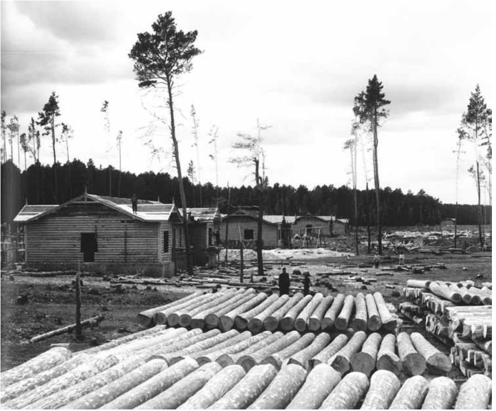
Railroad Construction on the Shchadrinsk-Sinarskii Line near Shchadrinsk, 1912.
