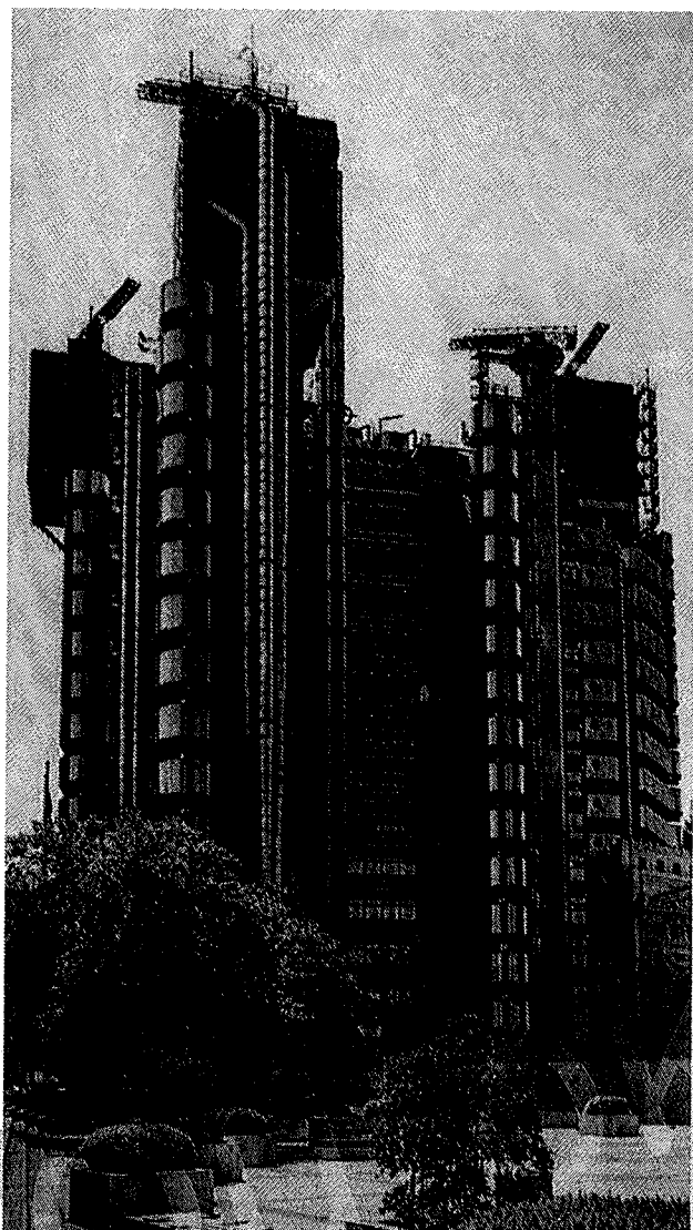
Figure 2:8. Lloyd's Building, London, completed 1986. Cladding in the austenitic Cr-Ni-Mo stainless steel 316 with HyClad® Linen surface finish.
