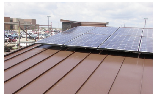
The Shakopee Environmental Learning Center from its construction to opening, with its wind generator and solar array.
