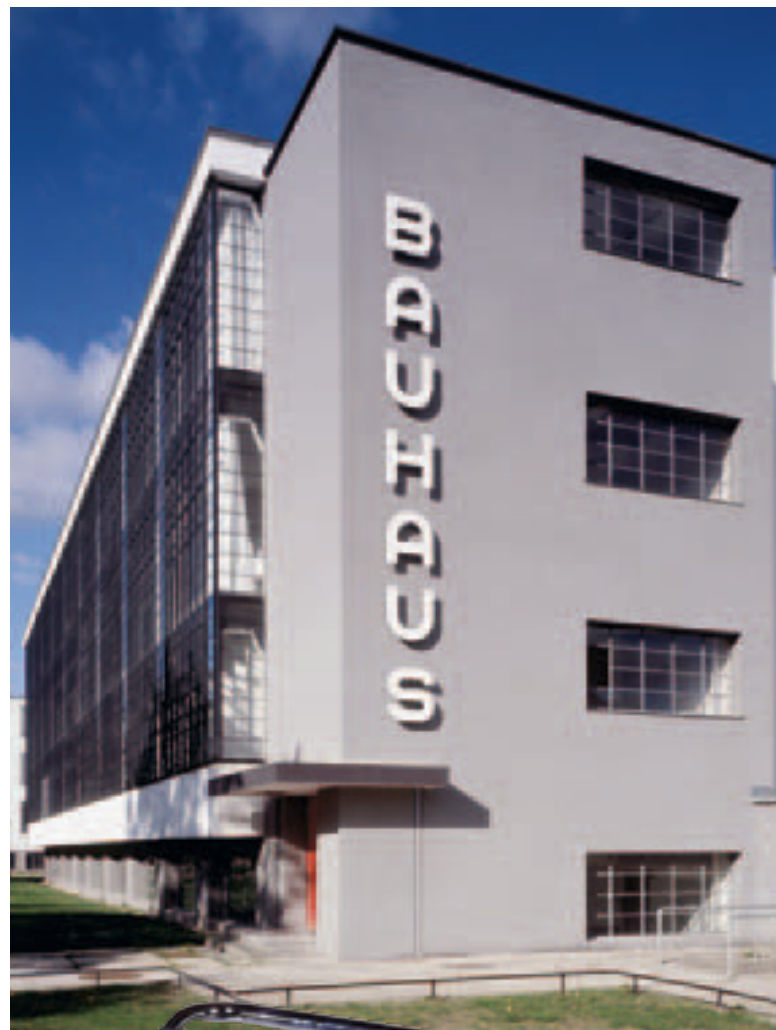
DESSAU BAUHAUS The concrete monolithic structure has glass curtain walls, which were a complete innovation in the 1920s.
