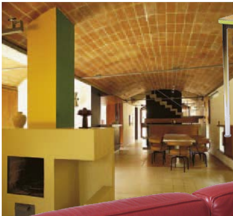
LA JAOUL, PARIS Designed by Le Corbusier, the vaulted brick ceiling unites the open-plan living and dining areas, providing a view through to the staircase.
