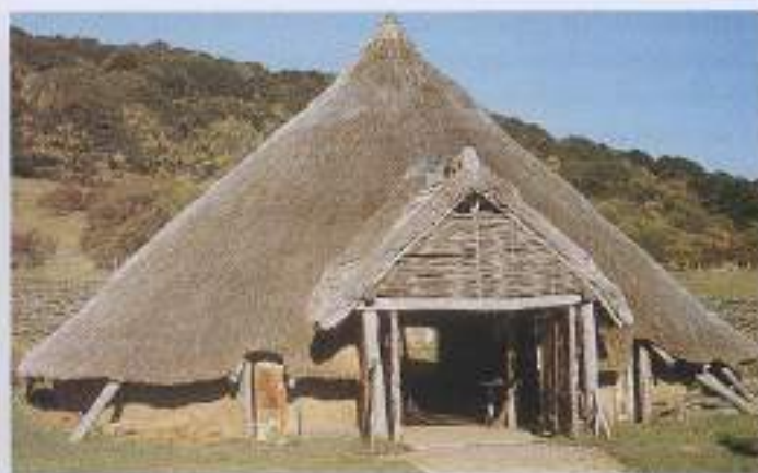
A reconstructed Iron Age farm. Farms like this were established in southeast Britain from about 700 bc onwards. This may have been the main or even only building; large round huts increasingly took the place of smaller ones. "Their houses are large, round, built of planks and wickerwork, the roof being a dome of thatch," wrote the Greek philosopher Strabo. In most of Celtic Europe huts were square.
