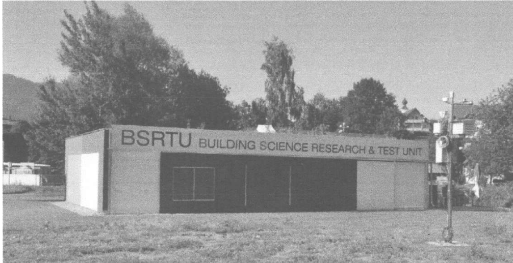
Figure 10. In situ measurements at BSRTU Outdoor Test Facility
