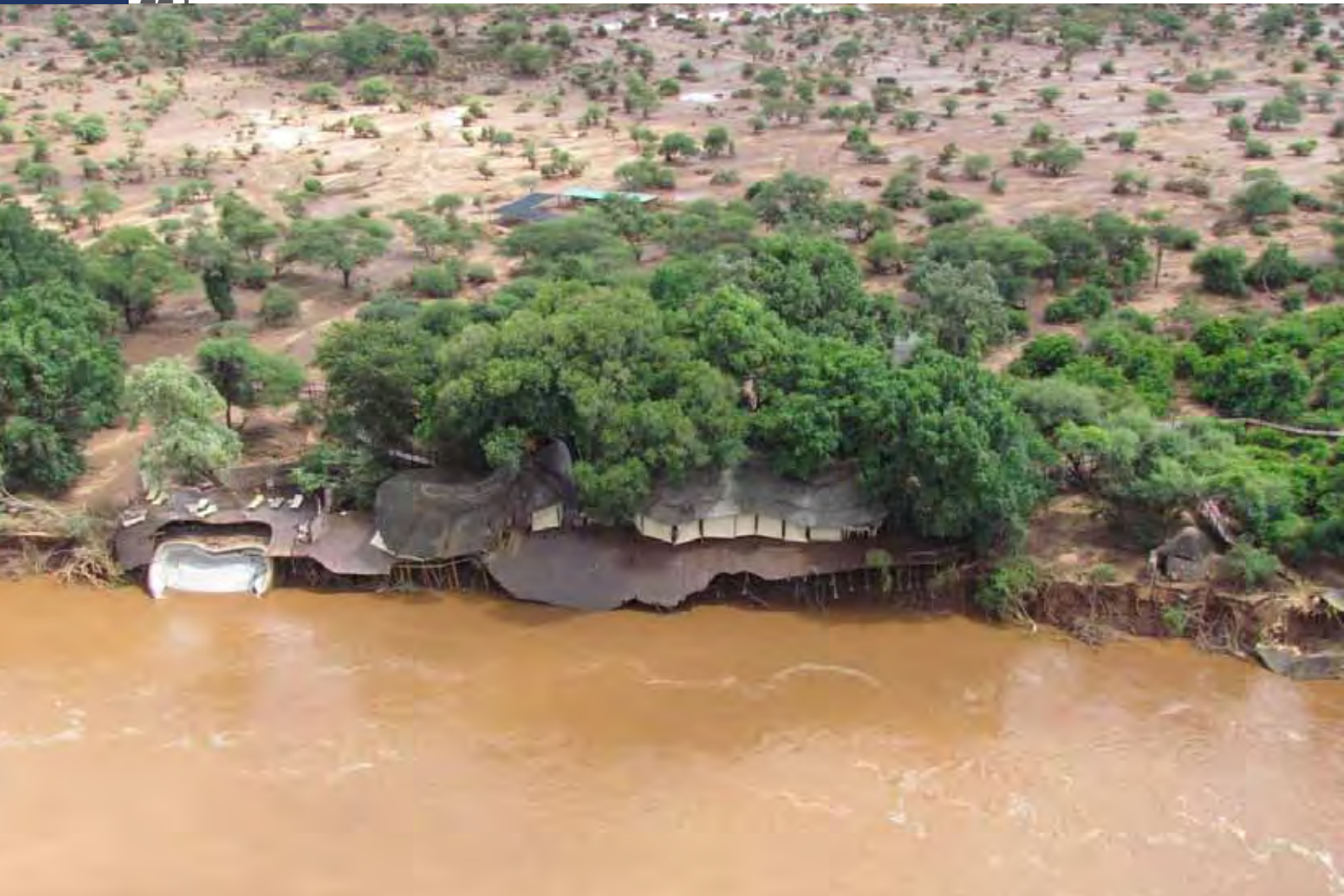
In an exceptional flood Pafuri Camp was destroyed. Should climate change impacts now be considered when awarding concessions? Photo: P.J Massyn.
